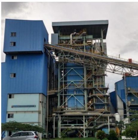
Gambar 1. Boiler CFB System di PLTU 3x10 MW PT. BEST Tanjung Enim
