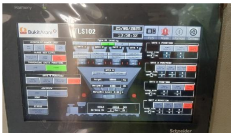
Gambar 2 Antarmuka HMI sistem Monitoring Gate TLS 102
