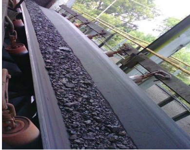
Gammar 1. Belt Conveyor Batubara PT. Bukit Asam
